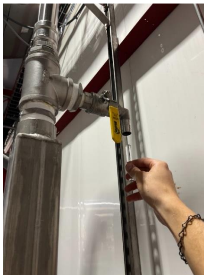
Figure 5: Rinse both the test tube and mixing bottle before testing
