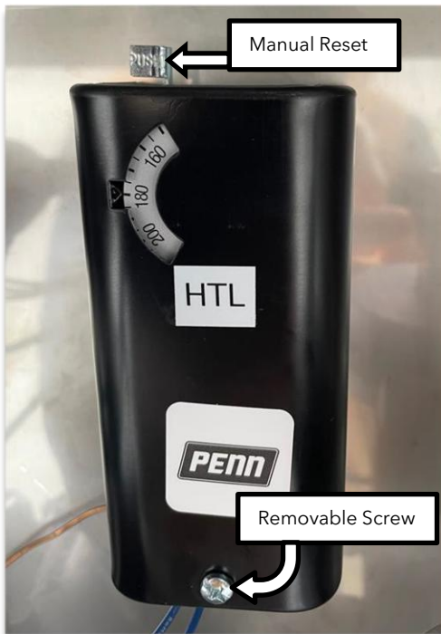
Figure 4 - High Temp Limit Switch w/ manual reset
