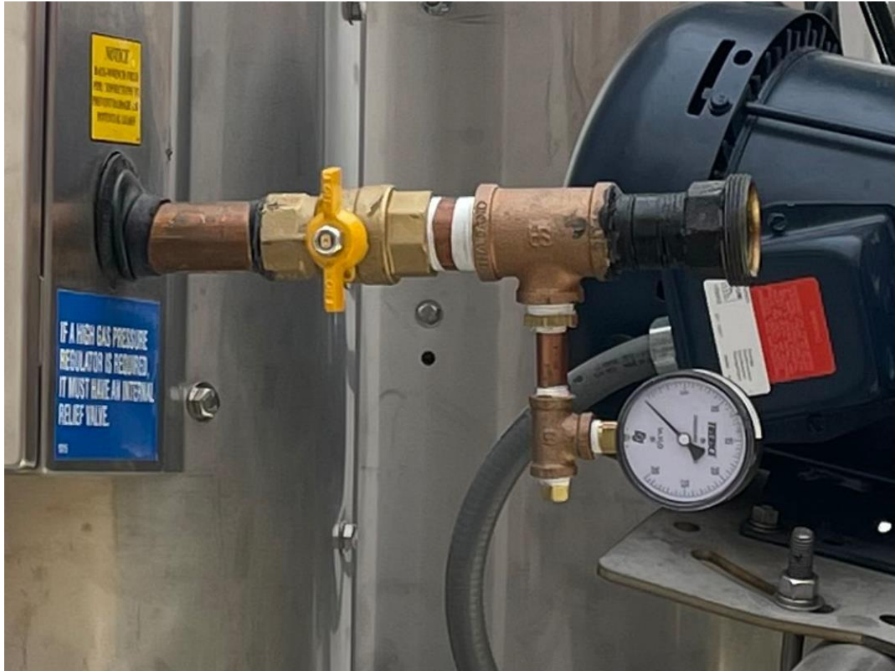
Figure 7 - External Gas Gauge Assy (P-HD-1021)
