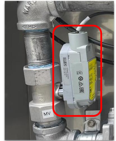
Figure 1 - Modulating Gas Actuator
