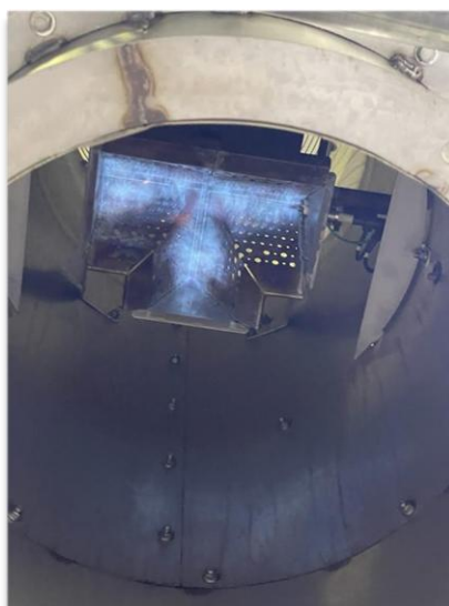
Figure 8 - Ideal Low Fire Flame Length
