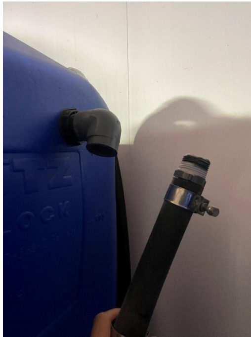
Figure 5: Unthread the hose barb from the elbow
