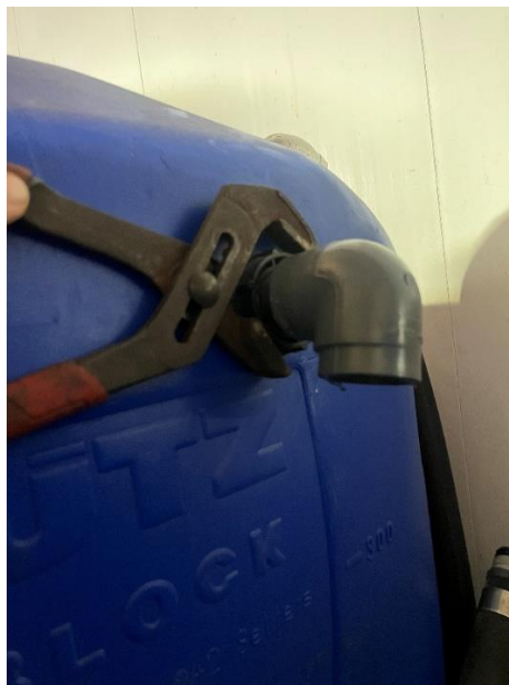
Figure 6: Tighten the bulkhead fitting with Channel Locks
