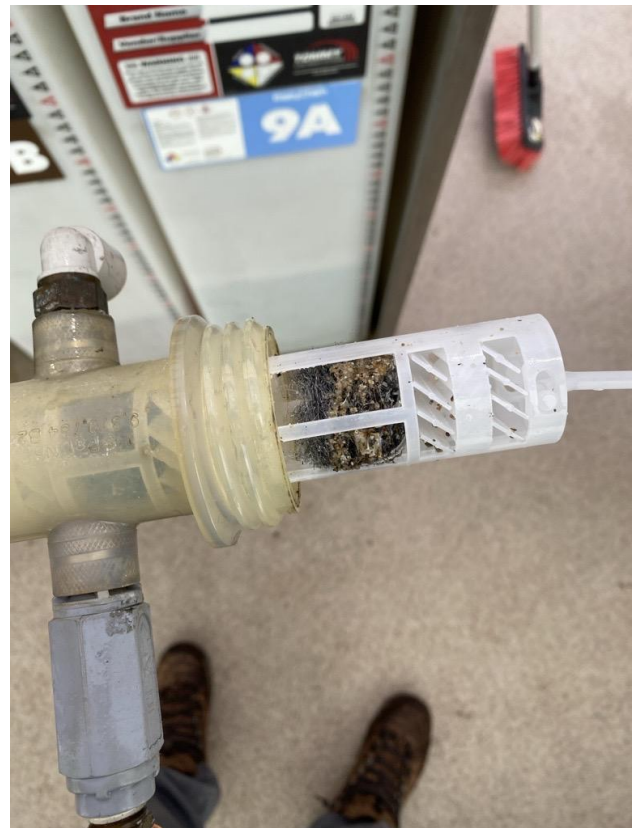
Figure 2 - Dirty Foam Generator Insert Pad
