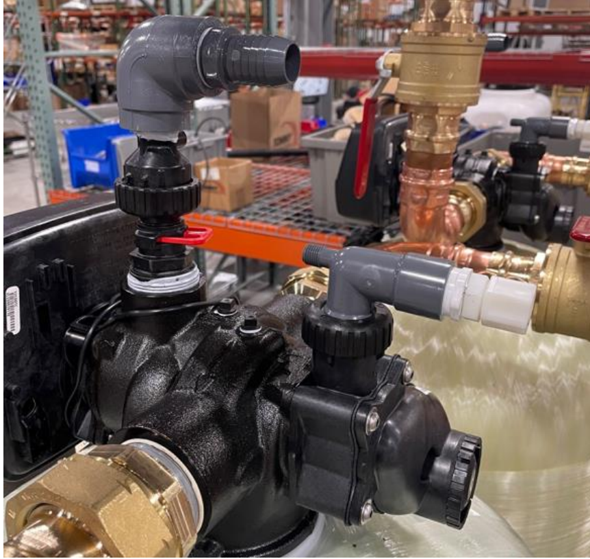
Figure 5 - Installed brine connection and drain fittings
