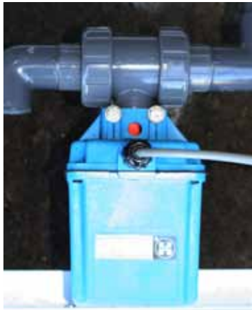
U/F Valve View Port: Red for Closed (top) Green for Open (bottom)
