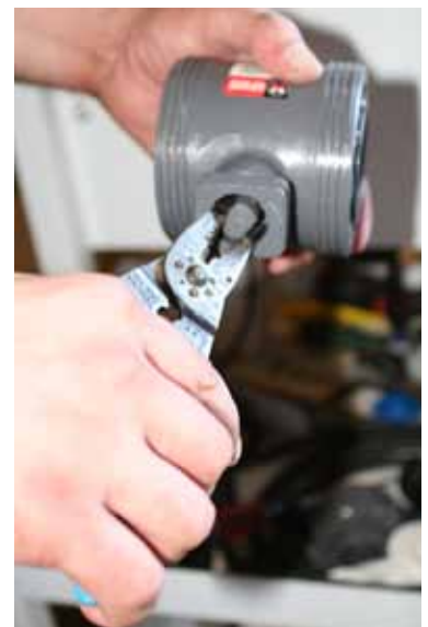
Valve needs to be turned so that it lines up with the motor collar
