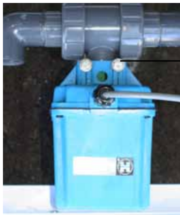
Use 7/16" wrench and socket (front and back) to disassemble valve from motor
