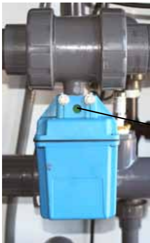
View Port on Recirc Valve: Green for open
